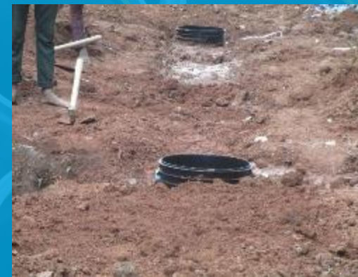
6. Back filling & Compaction
