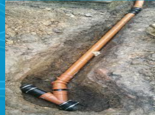
3. Sand bedding & pipe laying
