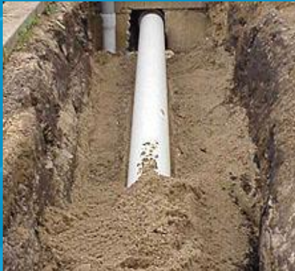
4. Sand filling upto crown of the pipe
